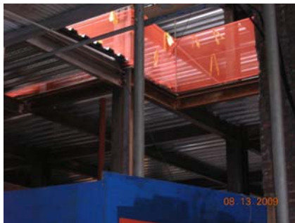
Figures F-2 and F-3: 40 Gold Street under construction
